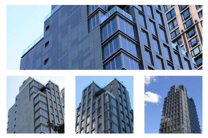
Manhattan's Upper EastSide new luxury building called The Isis Condominums was designed by FXFowle. The 28,000 square foot HPL rainscreen used the Plus5 attachment system. System Type: Vci.10 Panel Type: HPL Architect: FXFOWLE – New York Installer: Cardrona, Inc Completed: 2009
