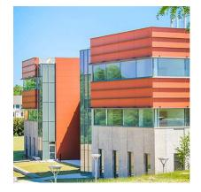
Cem5 fiber cement rainscreen is featured on a new building of the Harford Community College campus of Towson University in Northeastern Maryland (TUNE). IKON5 of Princeton designed the building using a custom sunscreen profile that was integrated with the Cem5 rainscreen wall.
