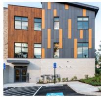
For the new 55,000 square foot facility known as "The Commons at Stanton Square" <u>Cladding Corp</u> provided a rainscreen solution incorporating CARAT and NOBILIS fiber cement panels from <u>SWISSPEARL®</u> and a VZ.10 rainscreen attachment system from partner company <u>ECO Cladding</u>.
