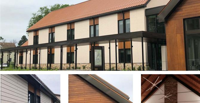
Ayers Saint Gross of Baltimore has designed the new Admission and Student Financial Services (ASFS) building at Grinnell University. Swisspearl® fiber cement and a wood grain HPL rainscreen were installed on an ECO Cladding sub-framing system.
