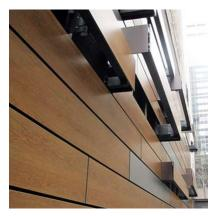
HPL panels and Plus5 attachment systems were married to create a unique facade on 1221 Avenue of the Americas. Various bracket sizes were used to achieve this 5,000 square foot wall. System Type: Vci.10 Panel Type: HPL Architect: Specter DeSouza Architects Installer: Advance Carpentry Const. Completed: 2009
