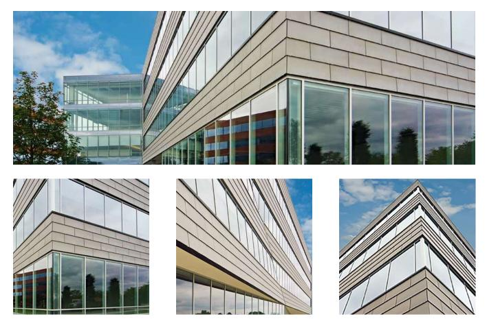
For this LEED rated installation at the Navy Yard in Philadelphia, our engineered Cem5 lap-siding is part of a revitalization that is both sustainable and long-lasting. Erdy McHenry Architecture were the designers. System Type: Vci.14 Panel Type: Cem5 Architect: emArchitecture Philadelphia Installer: Katzianer Construction Completed: 2009
