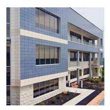
MGZA Architects created one of the first Ceramic5 projects in North America. The building is part of the corporate campus for the Wilmington-based water company with a focus on sustainable wall design and maintenancefree exterior cladding. System Type: Hci.20 Panel Type: Ceramic5 Architect: MGZA - Wilmington
