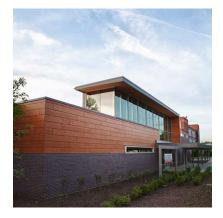
RDG Planning and Design of Omaha designed a HPL rainscreen wall featuring Plus5 substructure. An exposed fixing system was used and the depth accommodated fiber insulation. System Type: Vci.10 Panel Type: HPL Architect: RDG Planning & Design Installer: Boatman & Magnani Completed: 2012
