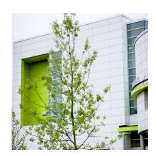
When designing the Academy of Advance Design and Technology, Amenta Emma Architects used Cladding Corp's Plus5 system on the HPL panels. The building features a variety of colors, including green, white and greys. The building also has a unique rounded front entrance.
