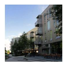
Designed by WDG Architects of Washington, DC, the new residential apartments on the HHMI campus incorporates the use of glass, metal panel and Cladding Corp's Cem5 fiber cement rainscreen cladding for the exterior skin of the project. The 22,000SF of Cem5 was installed using the Hci.10 visible rivet system, incorporating exterior insulation within the cavity to meet the project's R-Value requirements for the exterior envelope.
