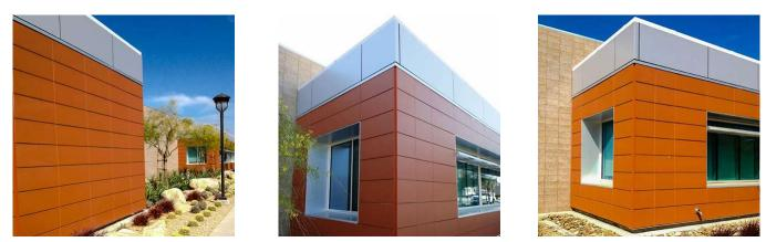
Terra5 was a natural choice for GKK Works of San Diego for the new Miramar College Service Center. The terracotta rainscreen added warmth and was the featured architectural facade material. Various features were added to create this energy-efficient building – including the use of green sunscreens. System Type: Hci.22 Panel Type: Terra5 Architect: GKK Works Installer: Sun Pacific Glazing Completed: 2011
