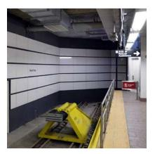
Cooper Carry of NYC designed the first new subway in NYC, with a Ceramic5 engineered porcelain stone cladding solution provided by Cladding Corp. Ceramic rainscreen systems are becoming more and more popular in the architectural design community. System Type: Vci.40 Panel Type: Ceramic5 Architect: Cooper Carry - NYC Installer: Judlau Contracting Completed: 2009
