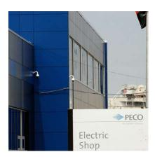
A 22,000 square foot HPL system used the Plus5 sub-framing for the re-clad of PECO Energy's Oregon Maintenance Shop. The corporate identity was embraced by blue and grey panels.
