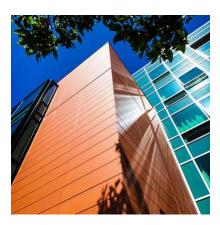
HKS – San Francisco designed Potrero Launch using Terra5 terracotta rainscreen. The new housing project used the terracotta panels along side bold window units to create a striking facade.
