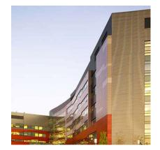
For this cutting-edge hospital project in Michigan, NBBJ Columbus selected a Ceramic5 rainscreen system along with wood laminate panels for the featured cladding on this facade.
