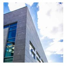
EYP Architecture & Engineering completed one of the most advanced stone rainscreen projects in the USA at SUNY Maritime College. The stone façade and precast was designed using Cladding Corp's PLUS5 attachment systems. System Type: Vci.44 Panel Type: Stone Architect: EYP Architecture Completed: 2012
