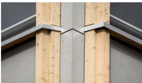
Visible mounting combined with the Closed Corner 90° system
