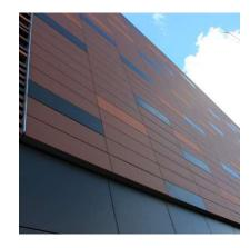
In preparation for Fall 2010 semester, installation of the University of Arkansas Garland Ave. Bookstore and Parking Garage is nearly complete with a Terra5 and Cem5 rainscreen and unique Terra5 baguette sunscreen.
