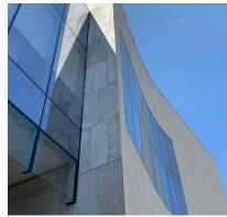
The center incorporates materials from different areas in Missouri including a dimensional limestone facade which is attached with ECO Cladding's Alpha Vci.41 concealed sub-framing system. The design by KCMO's Gould Evans reflects Missouri's geological characteristics. Installation of the limestone cladding was performed by Heitcamp Masonry of St. Louis.
