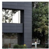
Open Studio Architects selected Terra5 terracotta panels to re-clad The Crossroads Office building in San Diego. The base of the building used a dark grey Terra5 panel and the upper levels of the building had an ACM system.
